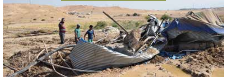
Demolition in the Jordan Valley in 2019.
