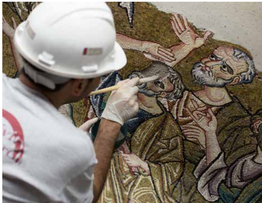
Restorer working on the wall mosaics of the transept.
