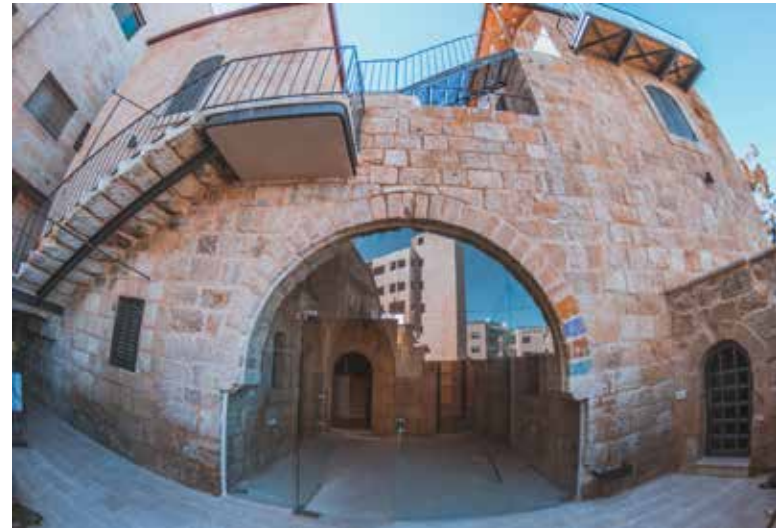
Renovating old houses in Ramallah.
