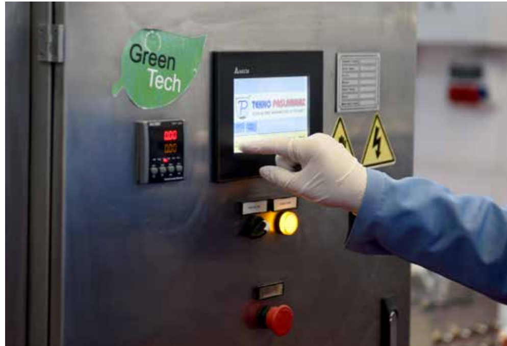
The rehabilitation and consolidation of Gaza Industrial Estate. Photo courtesy of UNDP/PAPP by Shareef Sarhan.
