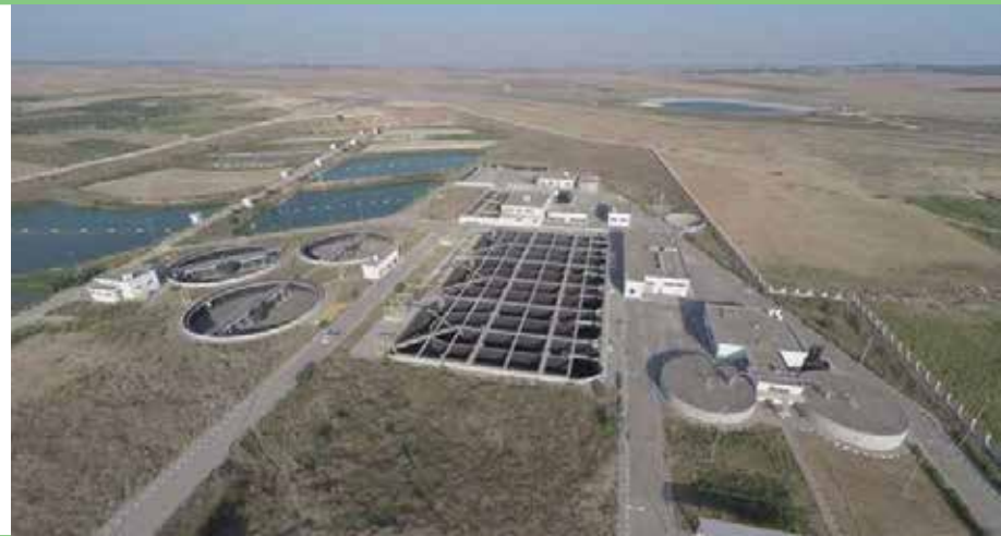
The new North Gaza Waste Water Treatment Plant.
