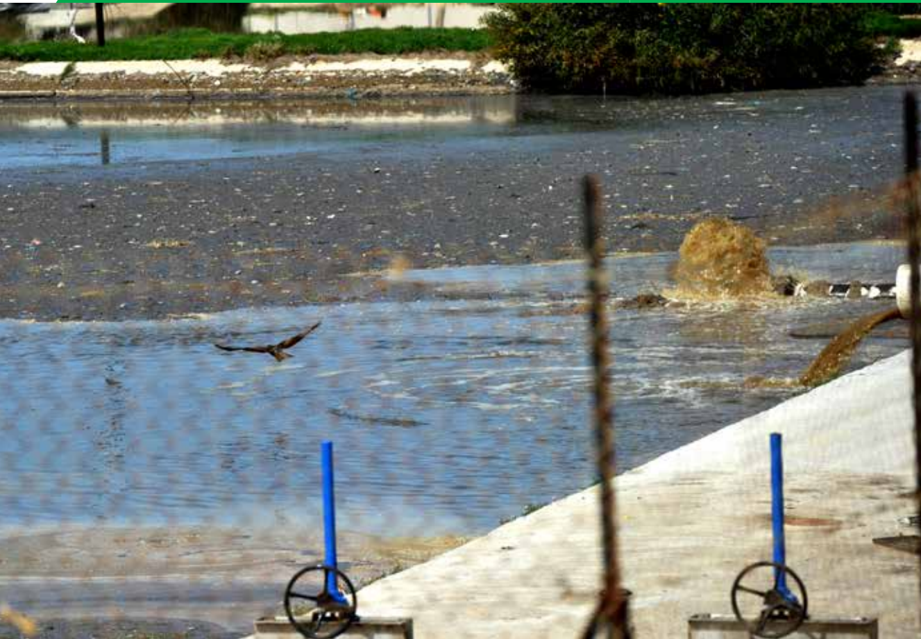
Sewage flood. Photo courtesy of UNDP/PAPP by Shareef Sarhan.
