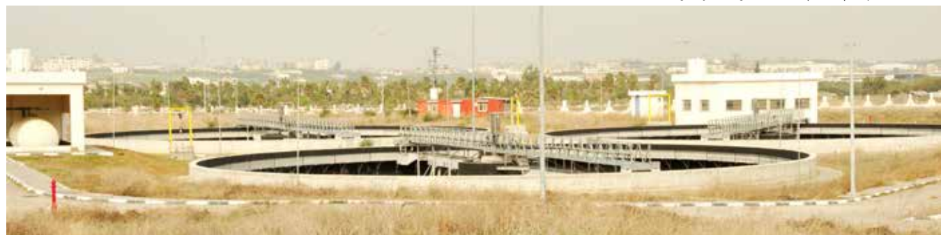
Northern Gaza Emergency Sewage Treatment (NGEST) Project.
