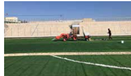
Installing artificial turf in the Jenin stadium.
