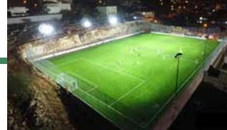
A renovated stadium in Sinjil, a Palestinian town northeast of Ramallah.
