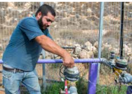
Farmer operating the treated wastewater subsoil irrigation system.
