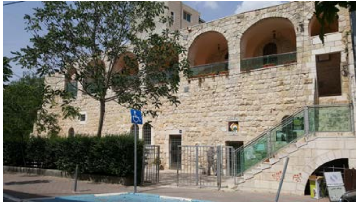
Ottoman Courthouse, Ramallah. Rehabilitation by Riwaq. Photo courtesy of the author.
