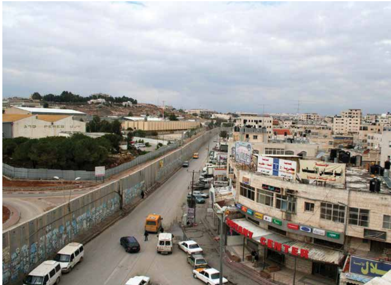
The Separation Wall cutting through Al-Ram main street.
