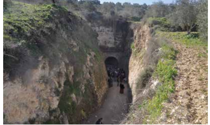
The Ottoman railway tunnel (Al-Kharq), Tulkarem.
