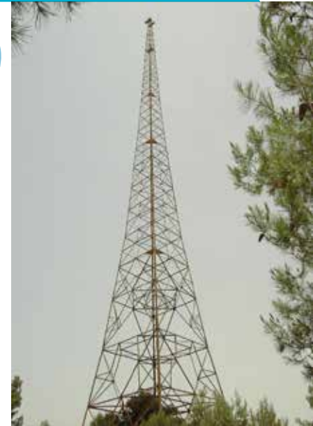
Irsal tower in Ramallah, the last remaining broadcast station of Radio Palestine. Photo courtesy of Wassim Abdullah.
