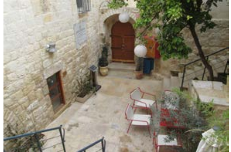
Syriac Hosh was rehabilitated in 2013 for adaptive reuse as a guest house in the heart of the historic center of Bethlehem.
